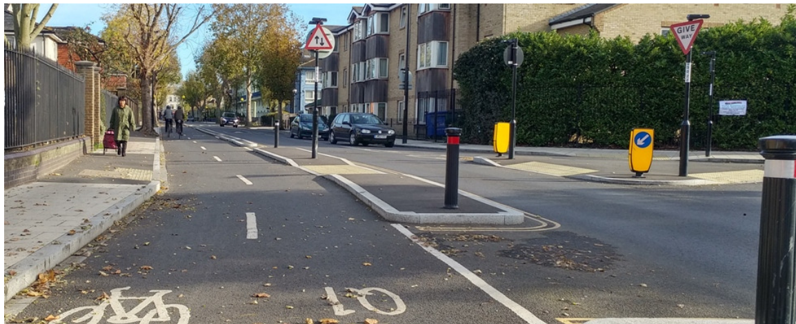
Figure 15 – recently completed Quietway 1
